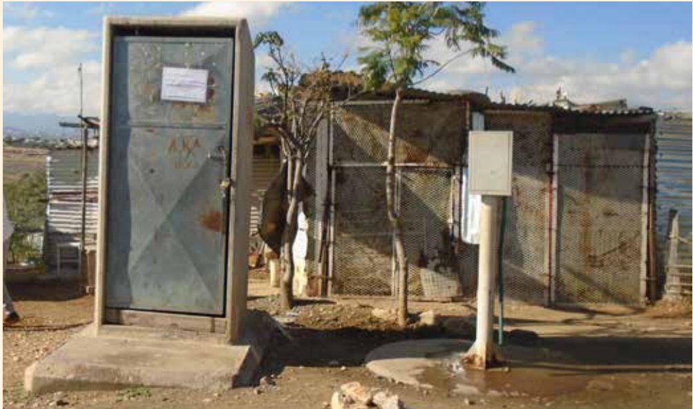
A shared flush toilet and communal water point in Havana.
