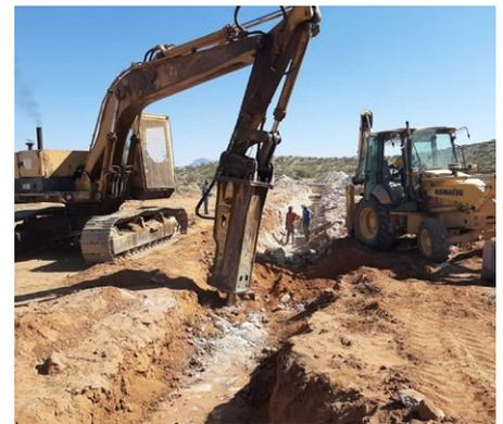
Karibib: Trench excavation for the laying of sewer lines. This is especially challenging in Karibib due to hard rock.
